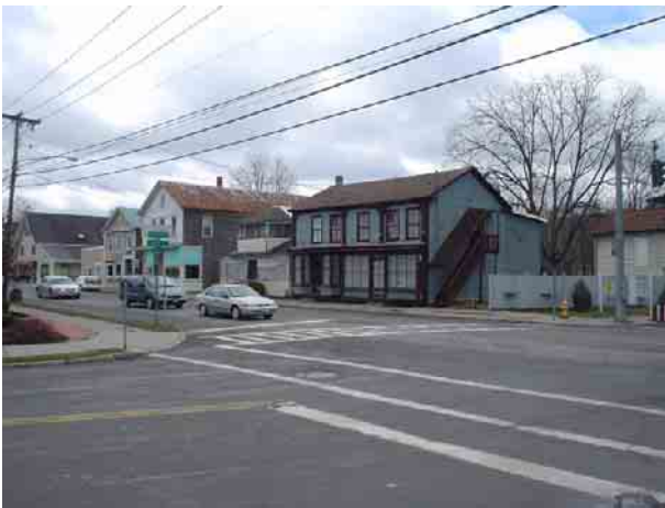
Figure 5.5 Village Streetscape (Before)
